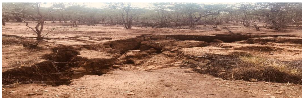
Plate 3.5-1: Erosion gully at Hoya business center
