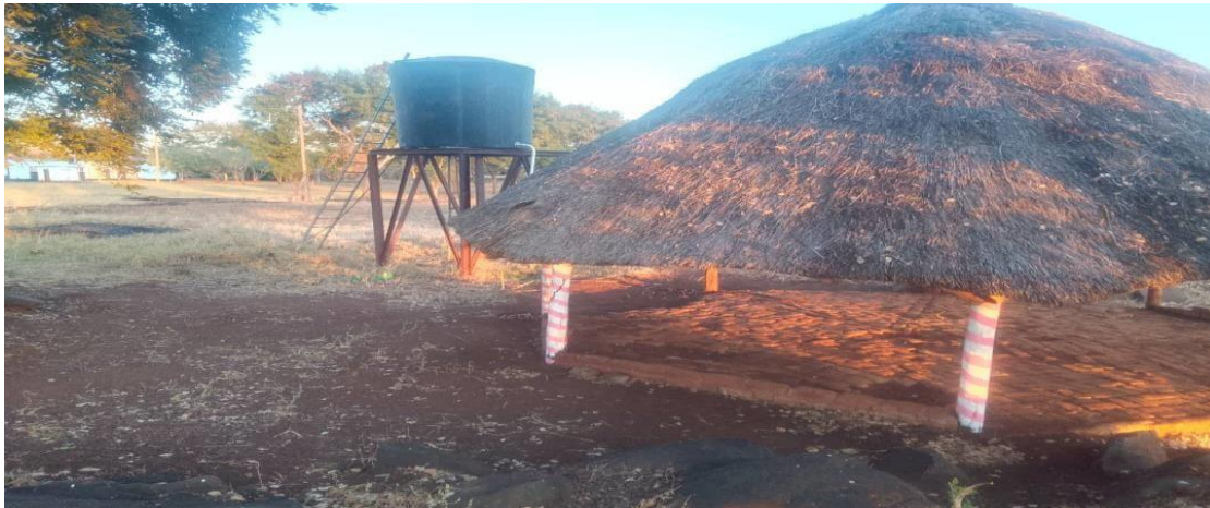
Plate 7.1-4: Gazebo and water tank for staff houses
