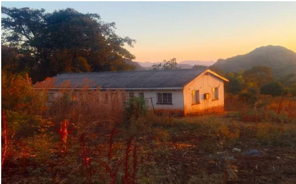
Plate 7.1-8: One of the 3 semi -detached Staff houses
